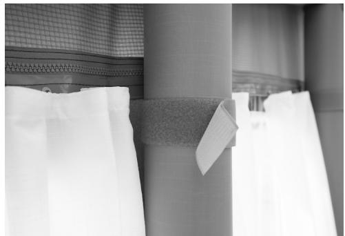
*After adjusting the height, attach the vertical supports to the PVC flap which is attached to the floor using the Velcro fastener which is located on the lower front section. This can also be used to create the required vertical tension for the front wall section.*
